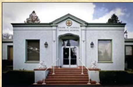
The Frank R Howard Memorial Hospital Community supported since 1928
